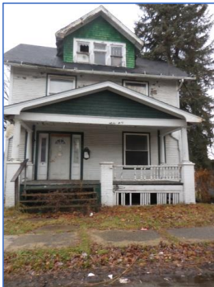
Vacant property on 5 th Avenue
